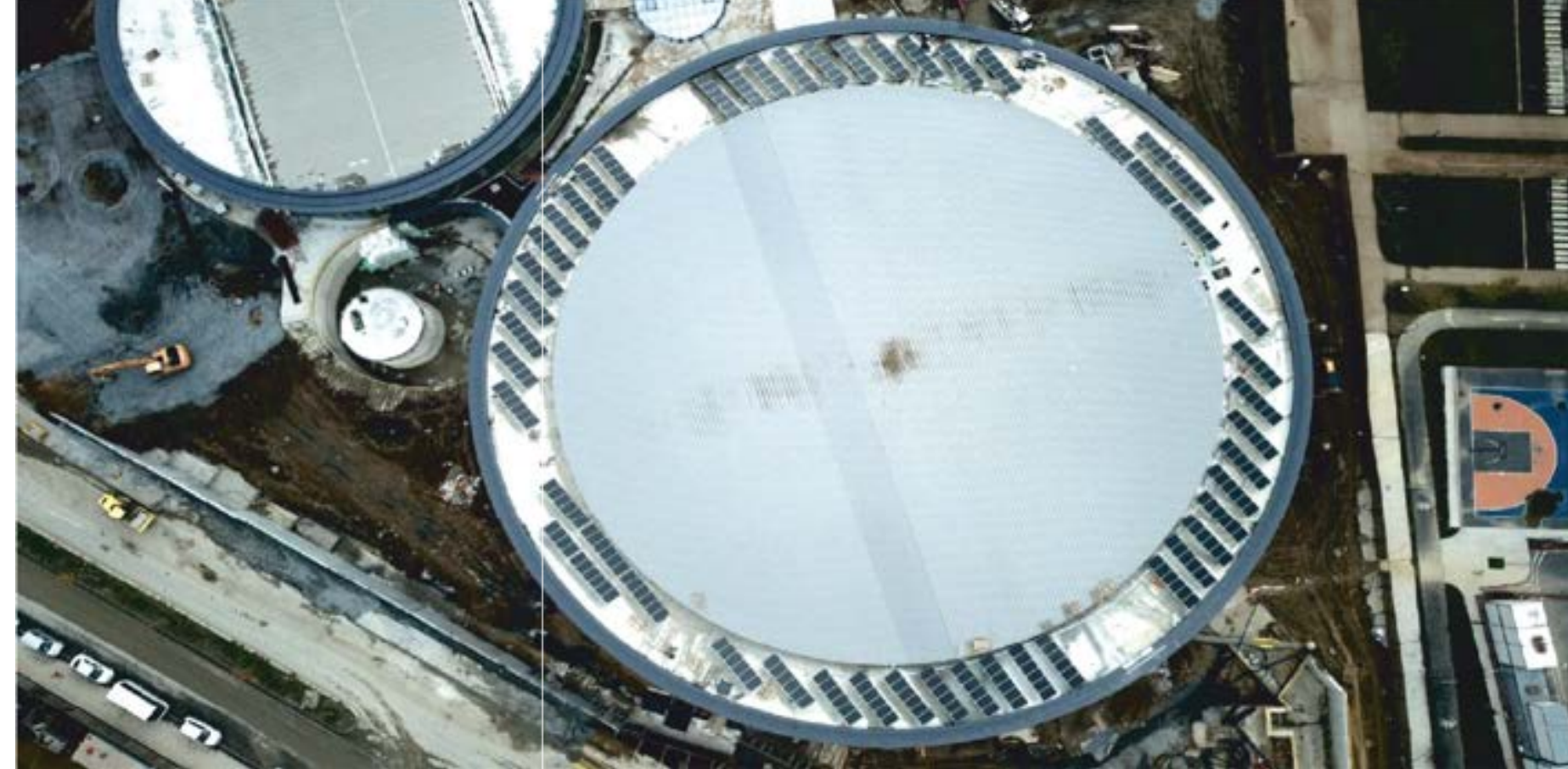
EMLAK KONUT / 100KWp / İSTANBUL / 2020
