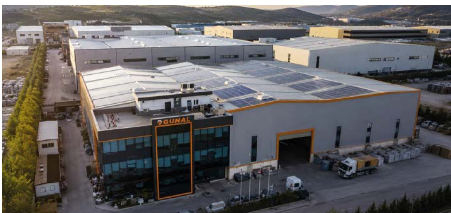
GÜNAL GEMİ / 304 KWp / 250 KWe / KOCAELİ / 2024
