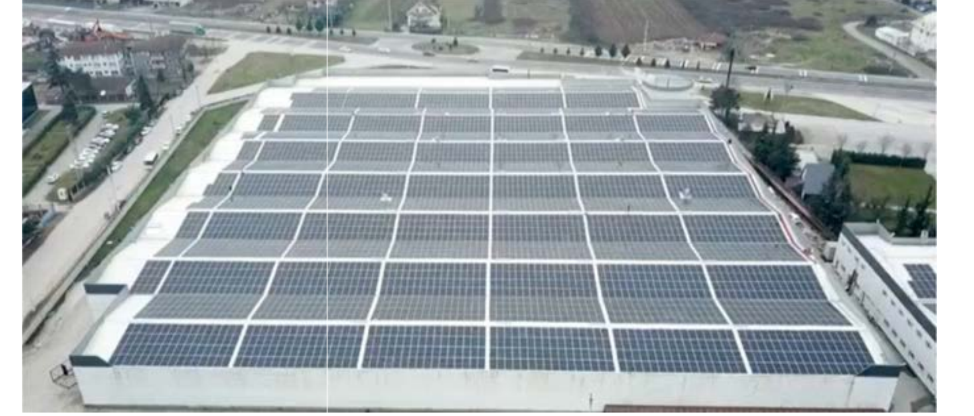
ÖRMA / 3051.4 KWp / 2460 KWe / DÜZCE / 2024
