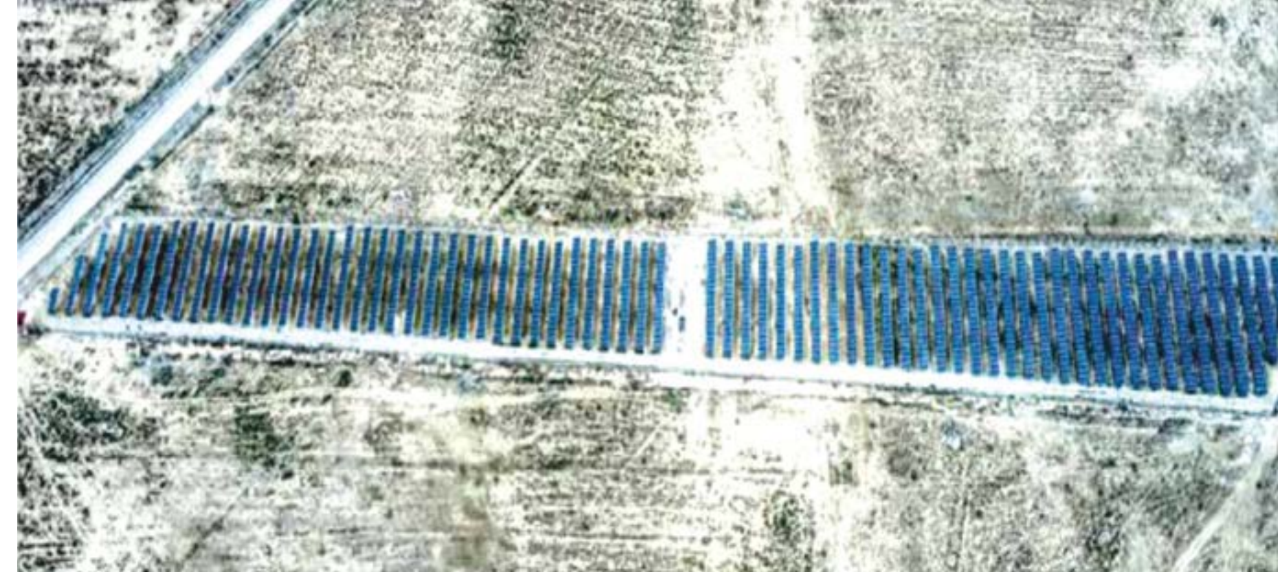
FİNA ENERJİ / 1.2 MWp / DENİZLİ / 2018
