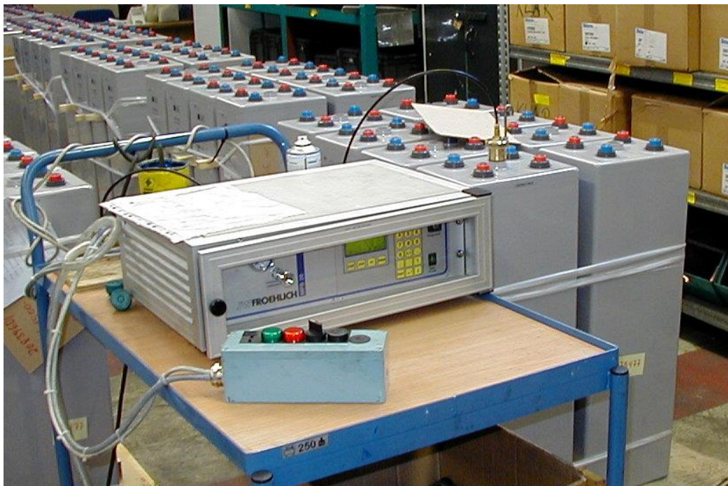
Figure 30 – Tightness test of 12 OPzV 1500 single cells.
