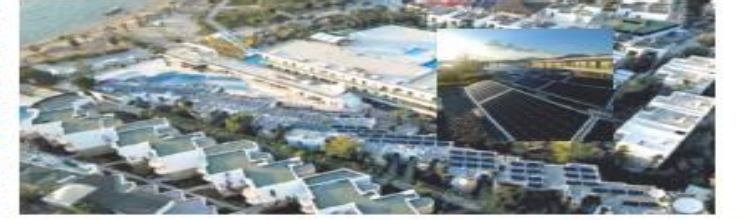
TROPICANA HOTEL /42kWp /MUĞLA/2019
